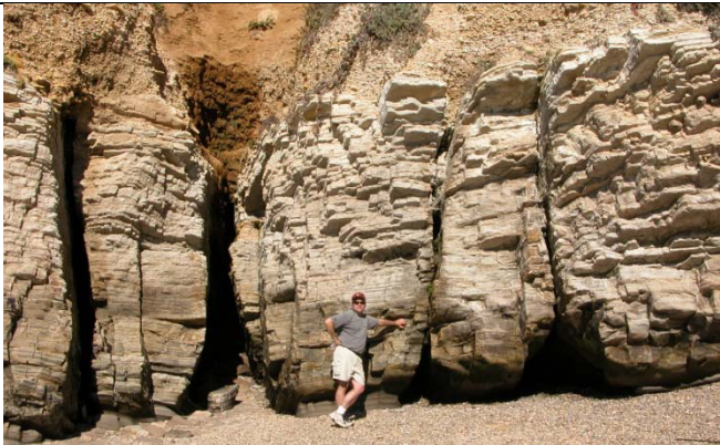
Figure I-22d. Large, throughgoing fractures at Point Buchon. These represent major pathways for fluid flow and provide vertical connectivity among fracture populations confined to smaller mechanical units.
